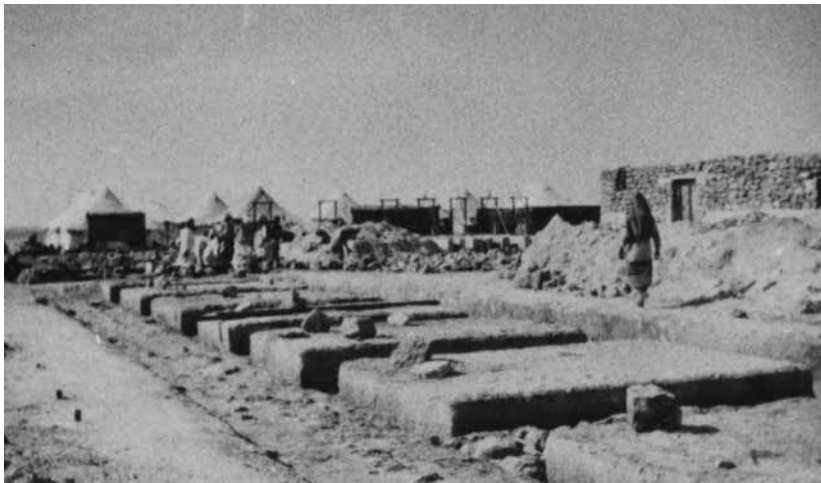
Laying the foundations for the rest house at Al Mahatta, Sharjah, 1932 ©Mackay Collection, His Highness Private Collection SM-NAC-1159
